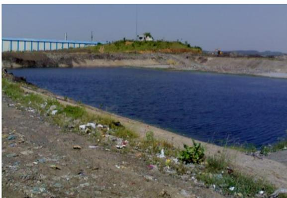
commissioning of new site, the waste started to transport here for processing as well as landfill. This site at village Kedarpur developed by M/s AKC Developers have disposal as well as leachate collection tank of HDPE liner to avoid ground water contamination.
